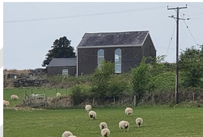
Above: Example of a traditional rural building, former Gerazim Chapel, Felindre
